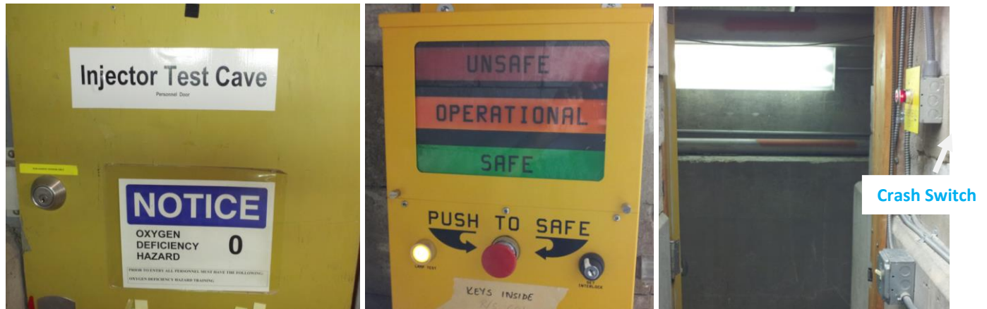
Figure 12 (Left) Exit door into high bay from Cave 1 near the electron gun (Middle) Run/Safe Box (Right) Crash Switch for exit. Run/Safe Boxes and Crash switches are at both the entrance/exit ways
