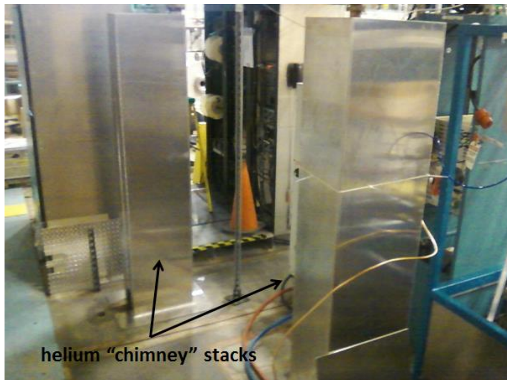
Figure 15. Two helium “chimney” stacks attached to rectangular penetrations in the ceiling of Cave 1. If helium gas is released inside the UITF enclosure, these chimneys will direct helium gas above the heads of staff members working near the electronics racks above Cave 1. Before energizing the QCM with high power RF energy, sandbags will be positioned at the base of each “chimney”.
