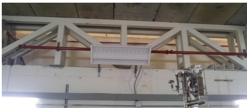
Figure 16: (top) Shielded elevated-roof section of Cave 2, which will be used for experimental targets, including cryogenic targets. (bottom) 5.6 m 2 Vent area beneath the elevated roof section of Cave 2, for lighter than air cryogenic gases to escape.
