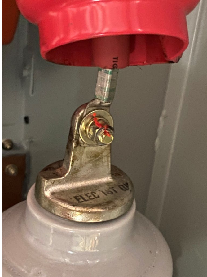
Figure E-21: Top of Phase A Surge Arrestor showing minimal heat discoloration on the front.
