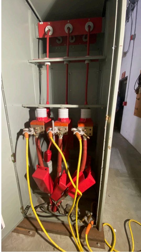
Figure E-18: View of BRK342 rear cubicle with protective grounds applied, as observed by the Board. Protective grounds were applied at the request of the Board (1/19/2023).
