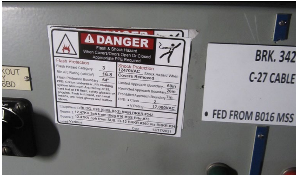
Figure 3-8: BRK342 Arc flash label shows two (2) sources, including MSS BRK75. It also indicates an arc flash boundary of only 64,” whereas it should be 59 feet.
