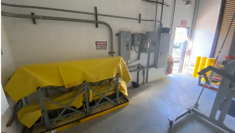
Figure 3-25: Battery bank at IR-2 Substation with insulating blankets over exposed energized terminals.
