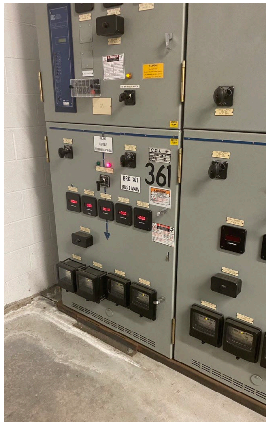
Figure 3-18: BRK361 in IR-12 is labeled as "Fed from IR-4," whereas it is IR-12 that feeds IR-4. The three arc flash labels have different values and do not match.
