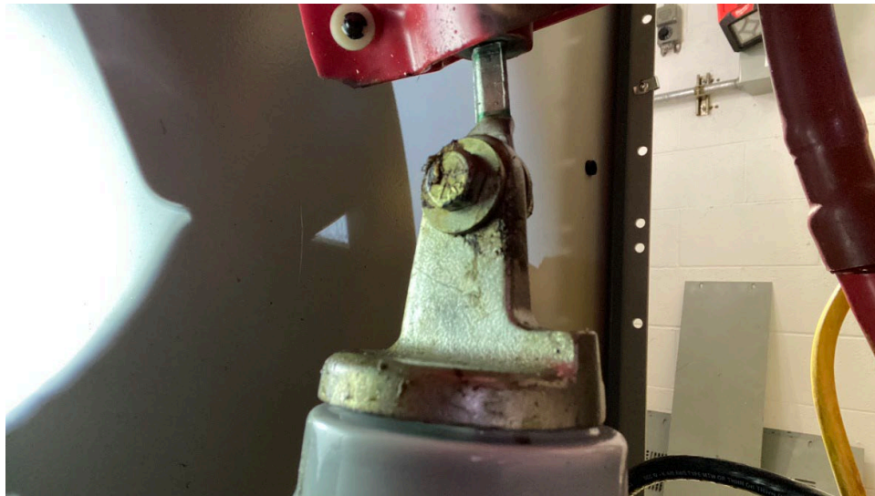
Figure 2-18: Rear view of the phase A surge arrester bolted connection showing deposits and slight thermal discoloration.
