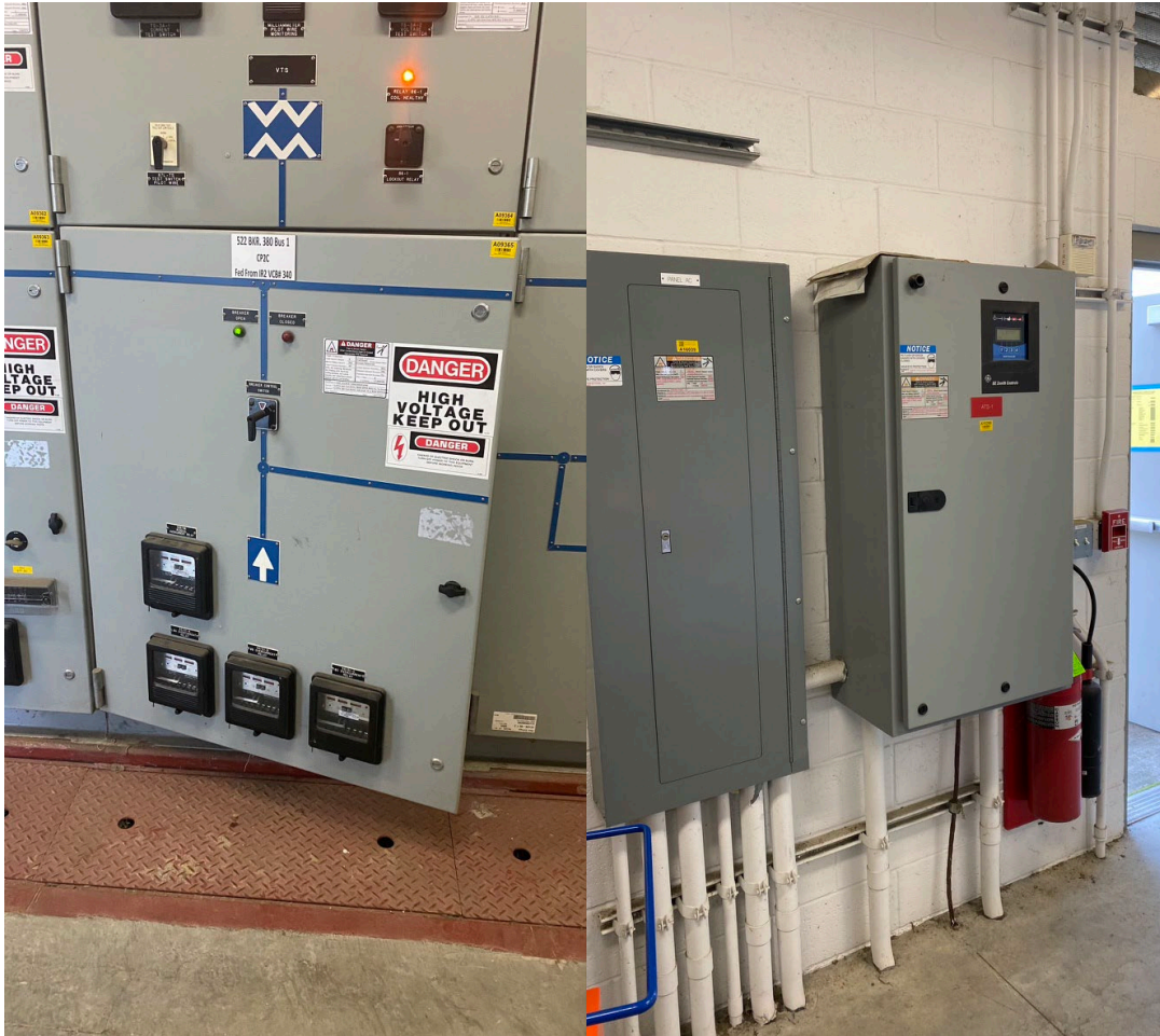
Figure 2-9: S522 Substation, BRK380 at left, ATS at right.
