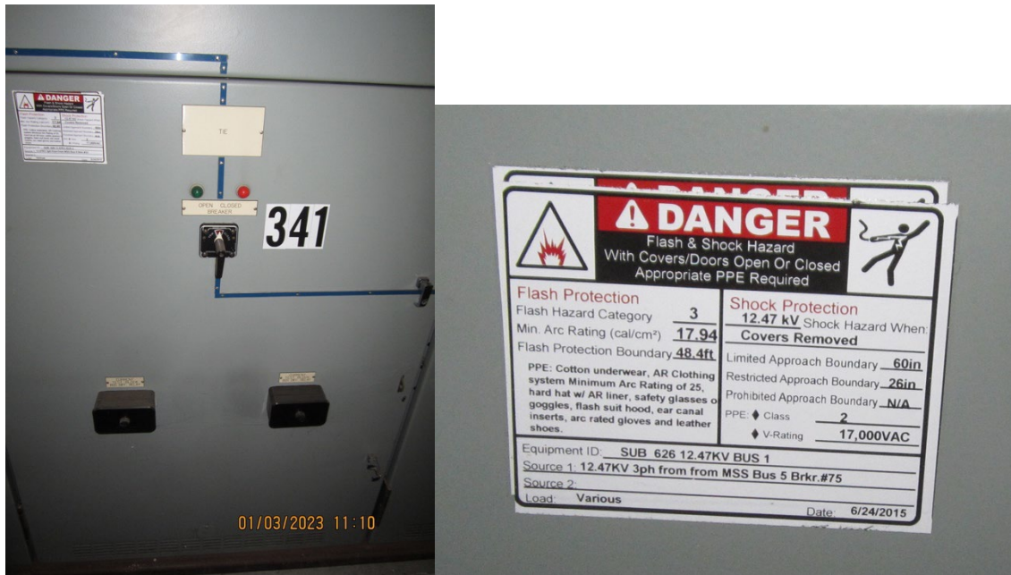
Figure E-8: BRK341 Arc flash label is still from 2015 and shows arc flash boundary of 48.4 feet.
