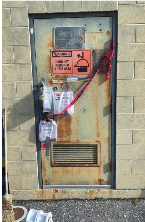
Figure 3-23: The main door to Building 626 / IR-2 Substation features dilapidated safety signs. The Danger sign on top has come off, and the label indicating minimum PPE for entry is peeled off and illegible.
