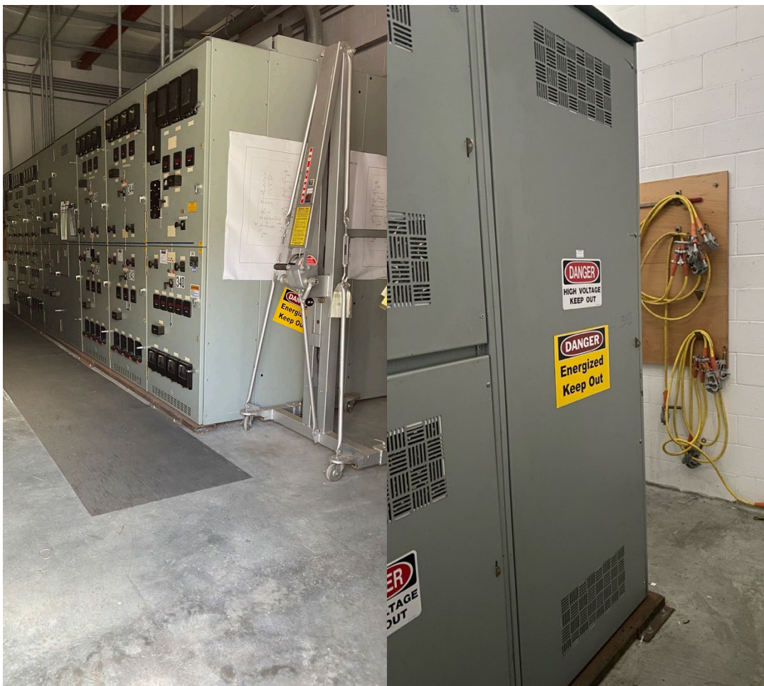
Figure 3-21: Temporary yellow magnetic Danger sign applied to IR-2 switchgear. The photo on the left shows the sign as found by the Board on the side of the gear. The photo on the right shows the sign applied to the rear door of BRK342 cubicle after the event for demonstration purposes by the HV Supervisor.
