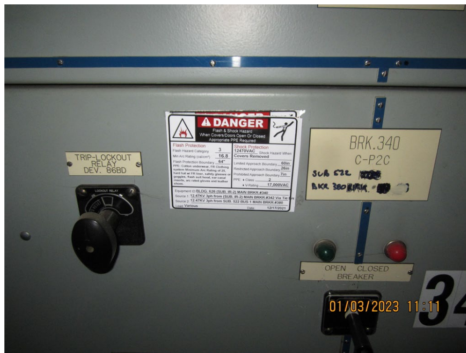
Figure E-7: BRK340 Arc flash label indicates an arc flash boundary of only 64", whereas it should be 59 feet.
