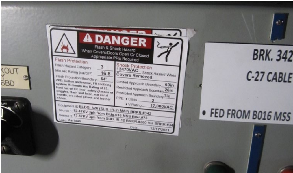
Figure E-6: BRK342 Arc flash label indicates an arc flash boundary of only 64", whereas it should be 59 feet.
