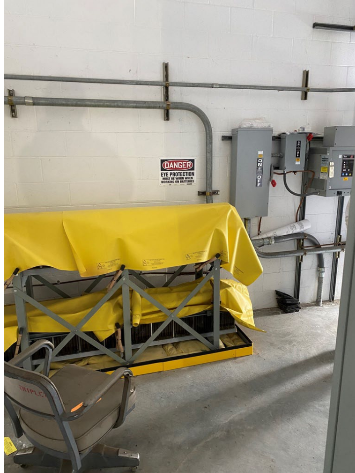
Figure E-4: IR-2 Substation 120 VDC Battery Bank was covered in insulating sheeting on 1/19/2023. Battery disconnect immediately adjacent to the right was opened by HVE1 on 12/27/2022.
