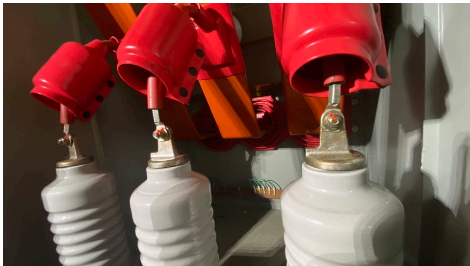
Figure E-20: All three Surge Arrestors with insulation boots lifted.
