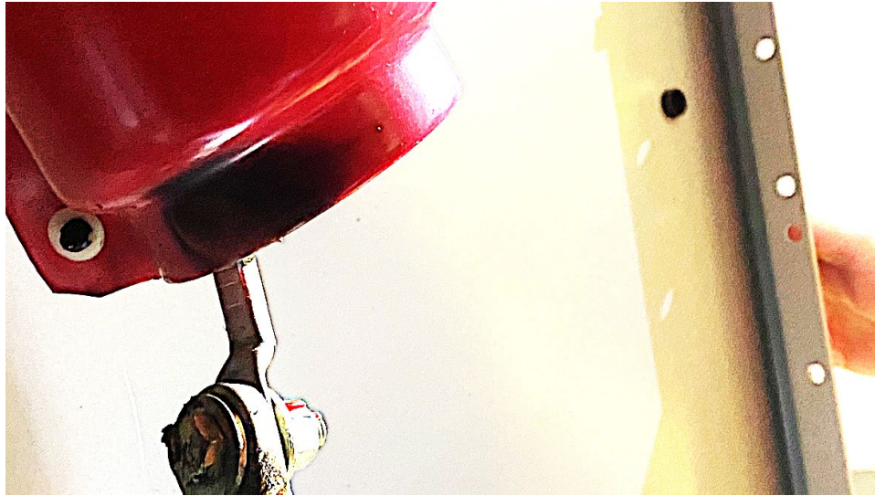
Figure 2-19: Rear view of the phase A surge arrester insulating boot showing some soot deposits.
