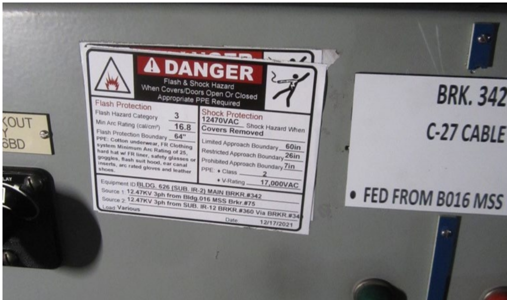
Figure 3-17: BRK342 Arc flash label indicates an arc flash boundary of only 64", whereas it should be 59 feet.
