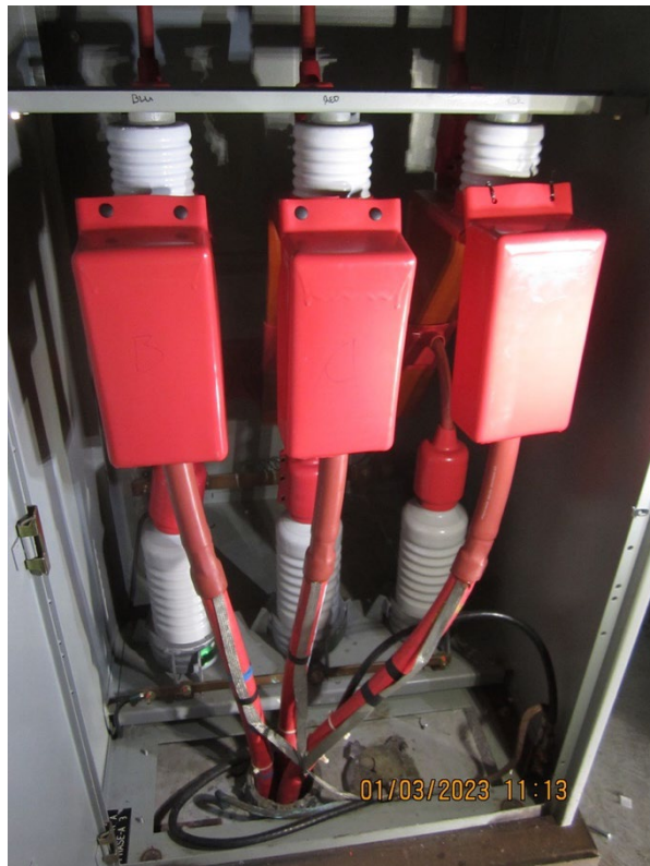
Figure E-17: View of BRK342 rear cubicle without protective grounds applied (1/3/2023).
