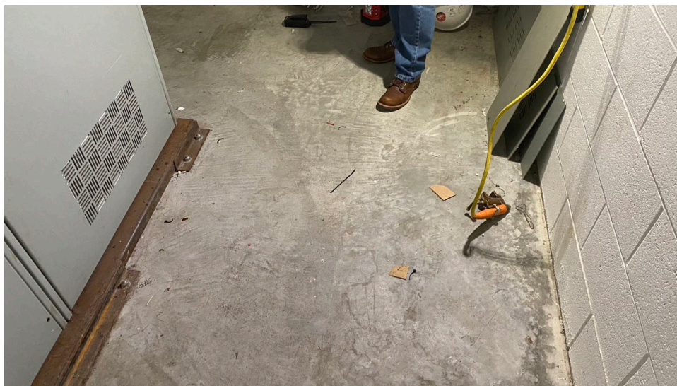
Figure E-12: Working clearance behind BRK342 was measured at 56". The ground clamp is for the discharge stick found hanging on the wall disconnect and staged for work by HVE3.
