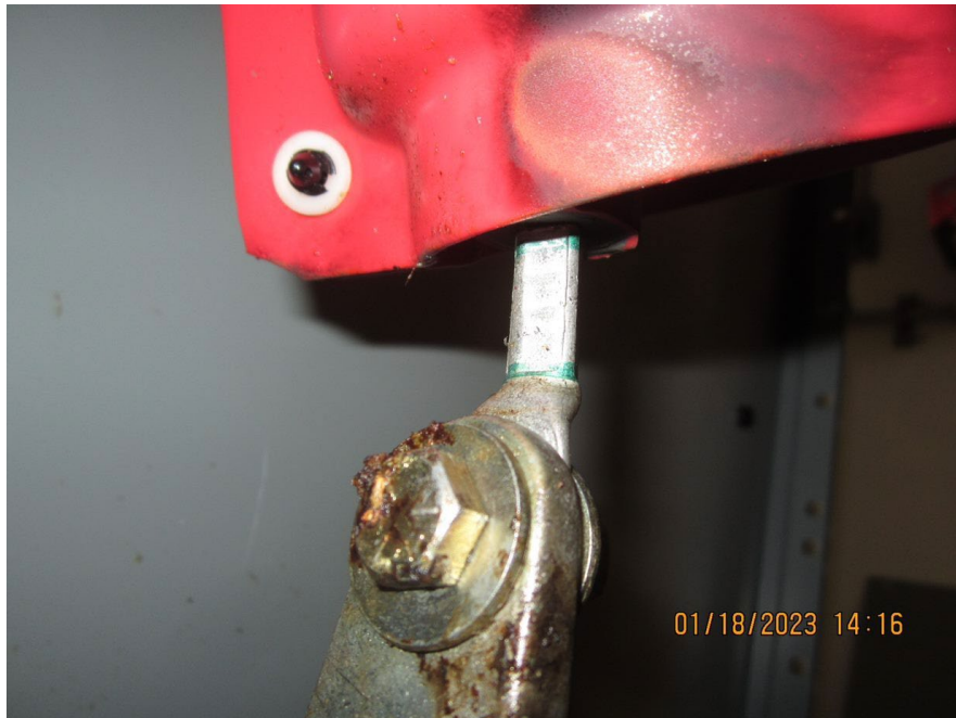
Figure E-22: Top of Phase A Surge Arrestor showing deposits on the rear. Also visible is soot and thermal damage to the insulating boot.
