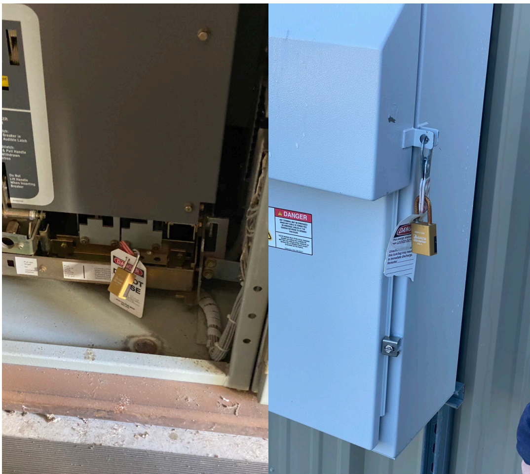
Figure 3-31: Examples of administrative locks applied with LOTO tags.
