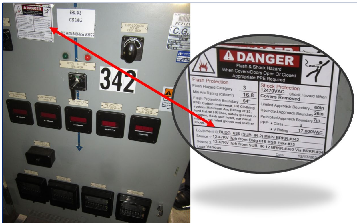
Figure 2-8: Arc flash label on BRK342 (B626/IR-2) showing BRK75 as a source.
