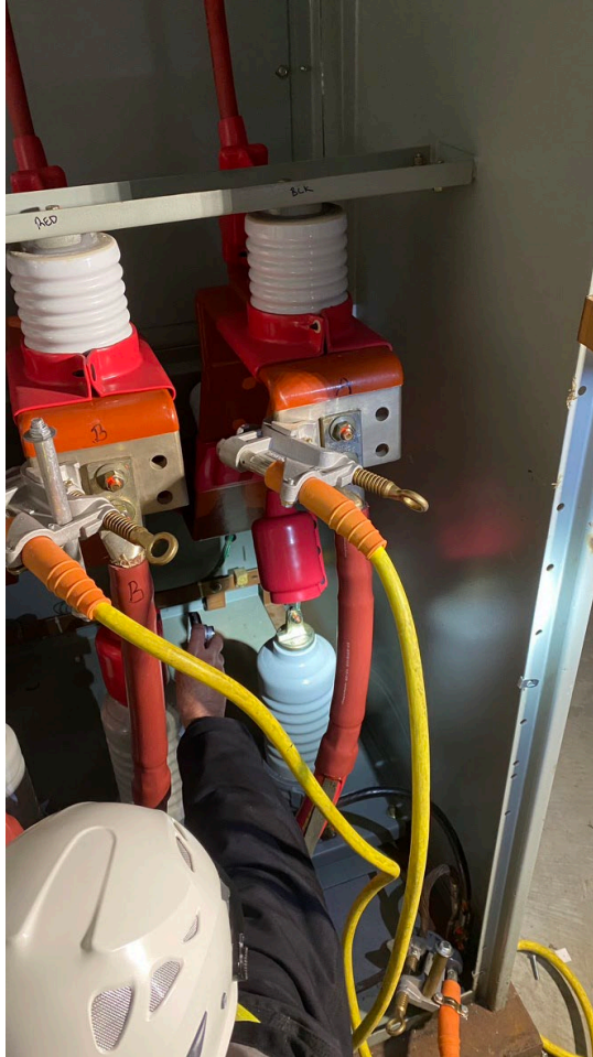
Figure E-19: Top of Phase A Surge Arrestor with insulation boot lifted, where HVE1 left hand made contact (location of shock).
