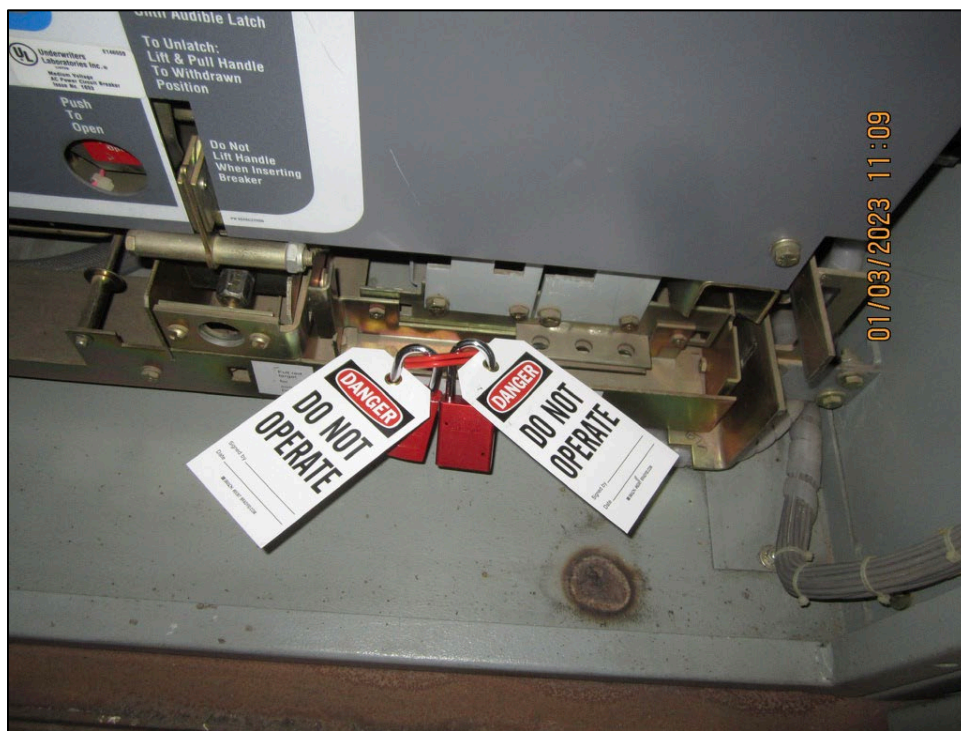
Figure 3-29: Group LOTO locks applied to BRK342 without Group LOTO tags and without any identifying information other than the number on the lock.
