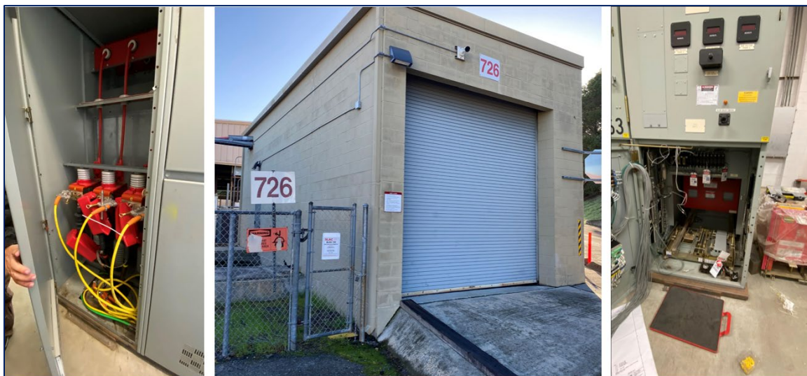
Figure 2-5: Building 726 with BRK360 racked out and grounds installed.
