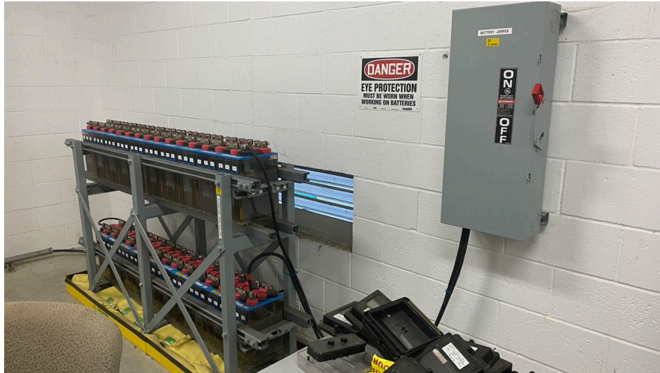
Figure 3-27: Battery bank at S522 Substation with exposed energized terminals.
