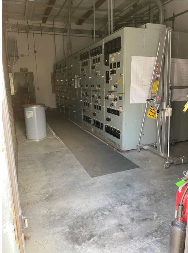
Figure E-2: IR-2 Switchgear, viewed from front door entrance. BRK340 is the closest and BRK342 is the farthest.
