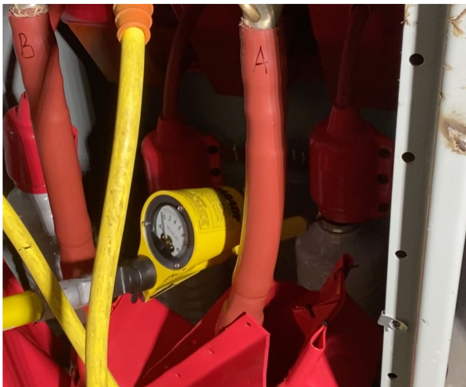
Figure 3-7: HV Supervisor demonstrating how the contact tester is used to lift the insulating boot to barely expose the top of the surge arrester on Phase A of BRK342 cubicle (already in an electrically safe work condition).
