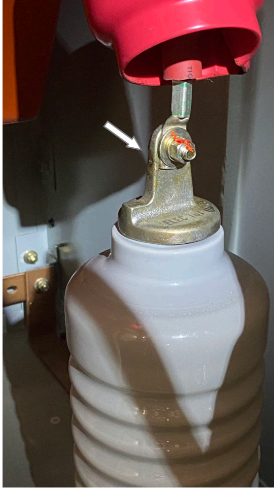
Figure 2-17: Front view of the phase A surge arrester bolted connection showing minor thermal discoloration.
