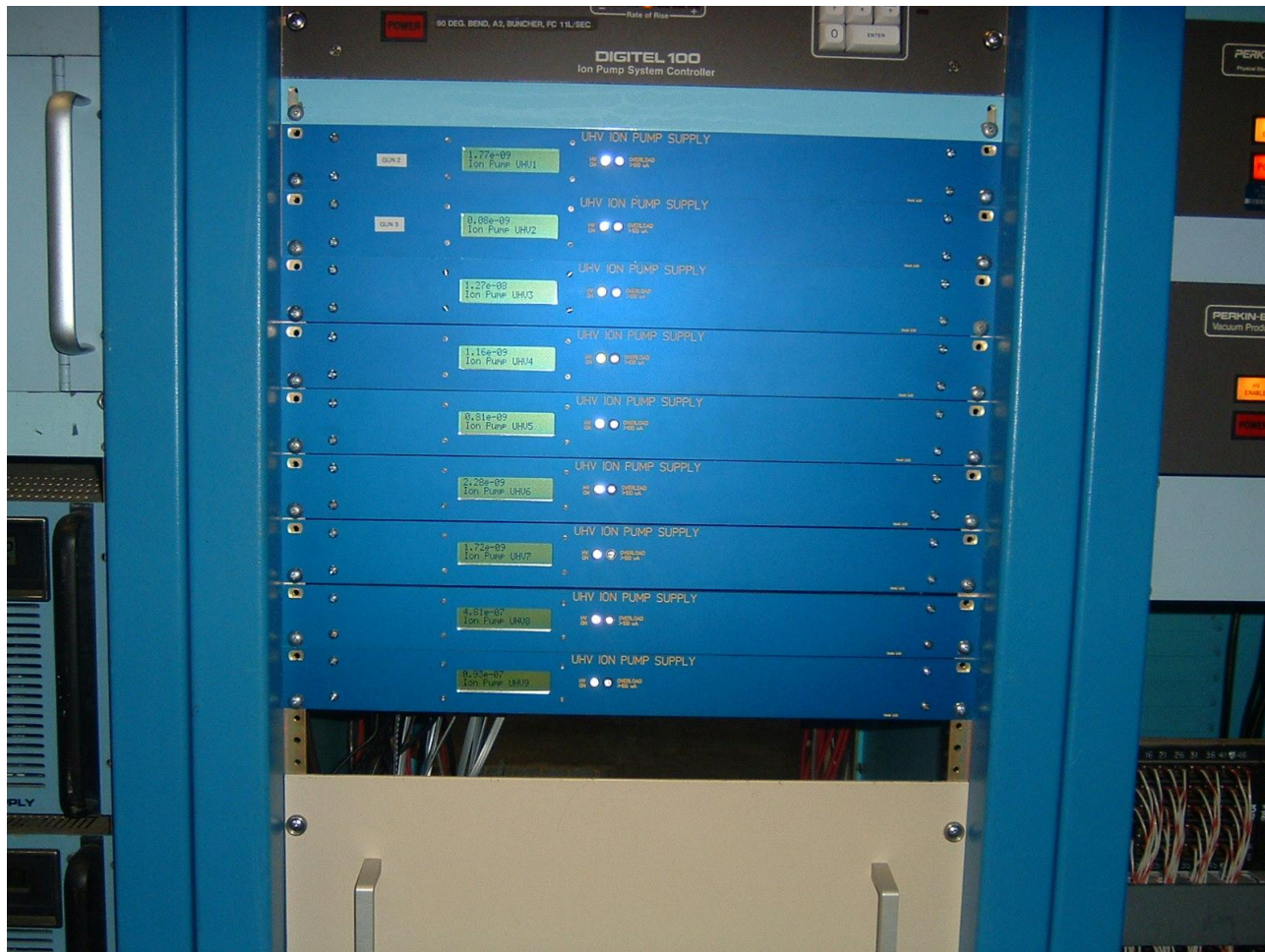
Figure 7. Nine supplies installed in 19" rack. All communicating over a single RS-485 network with the lab data acquisition system.
