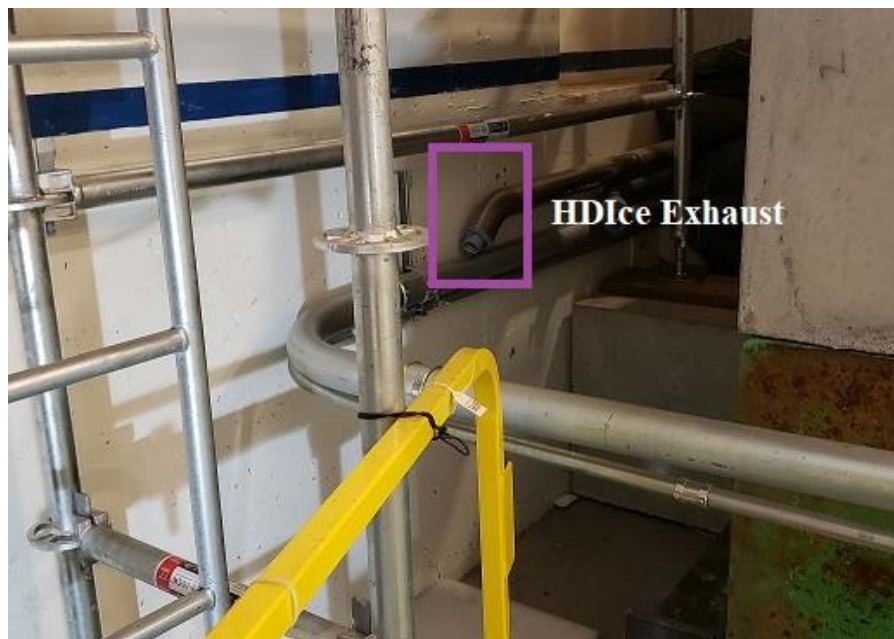
(Fig. 10: HDIce Gas exhaust port into the Test Lab High Bay)
