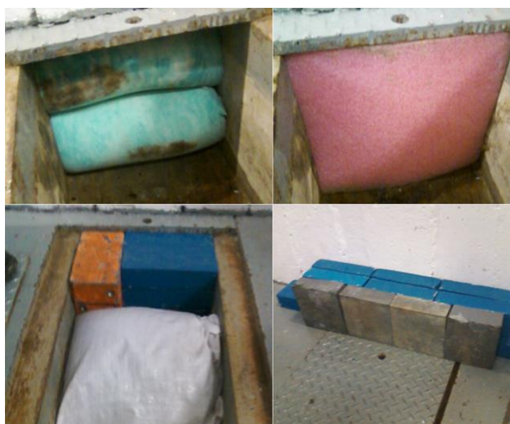
(Fig. 8: Sealed UTF cave cable trenches)
