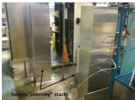
(Fig. 6: UTF Cave 1 roof Helium chimney stacks)
