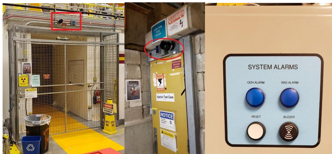
(Fig. 14: ODH alarm system indicators outside the UITF enclosure & within the Control Room)
