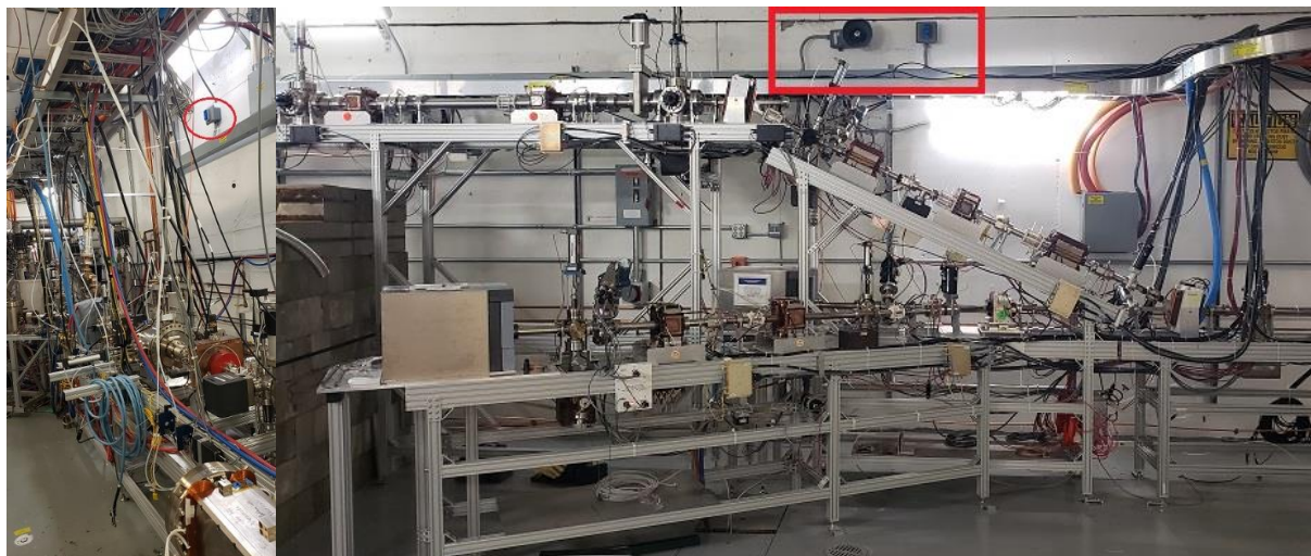
(Fig. 16: ODH Warning Strobes & Sirens internal to the beam enclosure)
