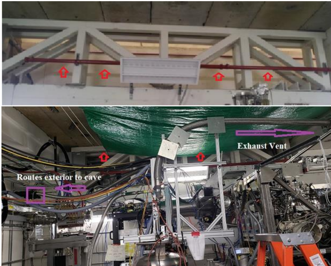
(Fig. 9: HDIce Gas Venting [internal to beam enclosure] | Purple = Target Boil off / Red = Catastrophic loss)
