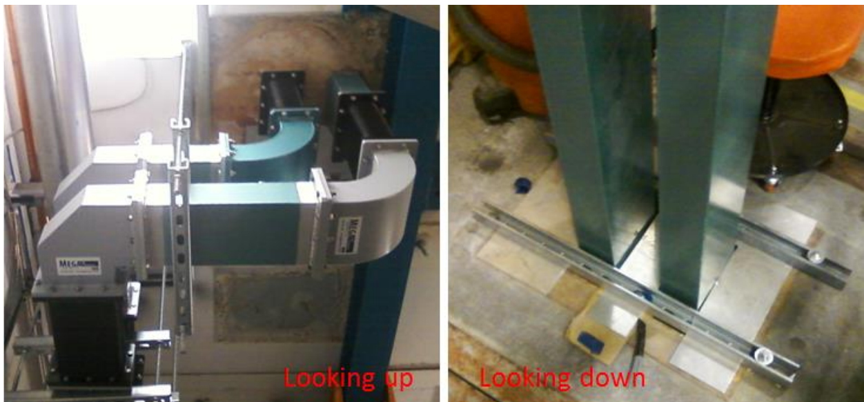
Figure 4: Steel plates covering penetrations in Cave1. Cables pass through the penetrations linking the electronics racks and beamline elements.
