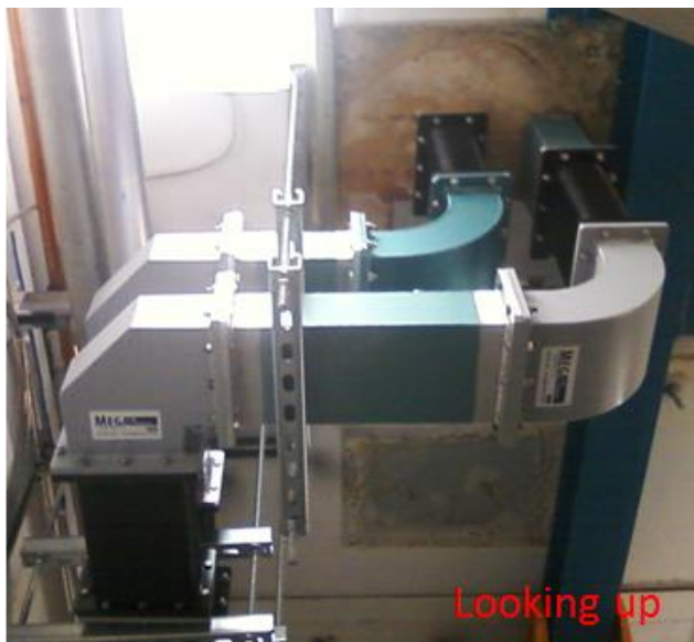
Figure 4: Steel plates covering penetrations in Cave1. Cables pass through the penetrations linking the electronics racks and beamline elements.
