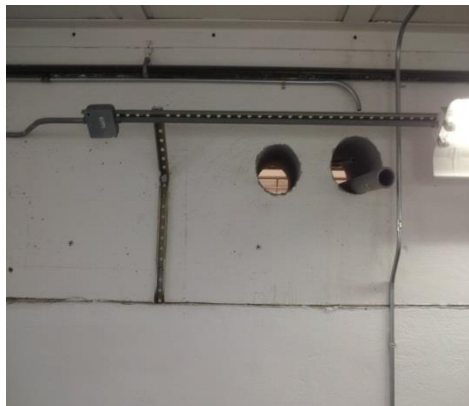
6" Vents, West Wall
