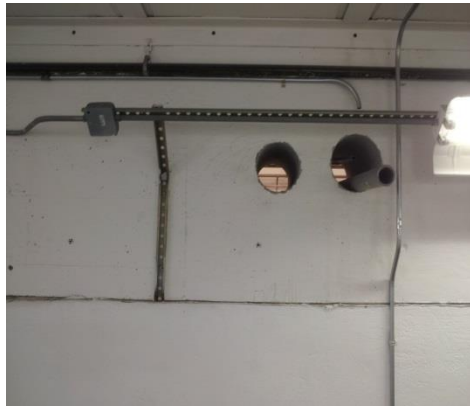
6" Vents, West Wall
