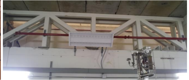
Figure 9 (Left) Shielded elevated-roof section of Cave 2, which will be used for experimental targets, including cryogenic targets. (Right) 5.6 m 2 Vent area beneath the elevated roof section of Cave2, for lighter than air cryogenic gases to escape.
