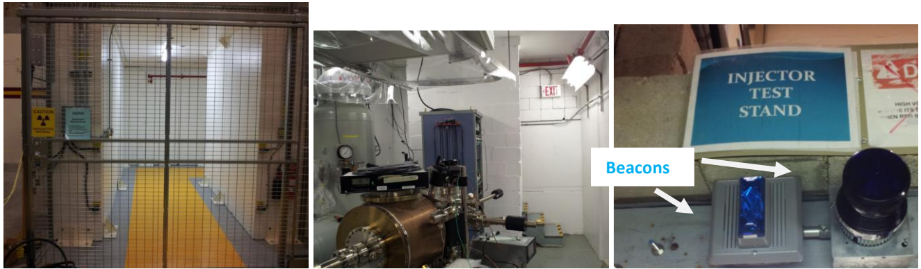
Figure 6 (Left) Main entrance/exit from high bay area through the labyrinth of UITF (Middle), Secondary exit into the high bay from the southern-most location of the keV section. Both doors have Personnel Safety System interlocks and emergency exit switches on the nearby walls (Right). Beacons exist at both entrance/exit ways
