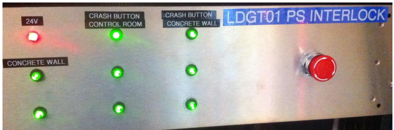
Figure 5: Cathode magnet power supply interlock box in the GTS Control Room (Rack GL01B15) The PSS Interlock chassis (shown in Figure 5) displays the status of the power supply interlocks. All interlocks must be green to be able to turn the supply ON. Figure 6 shows the power supply control
