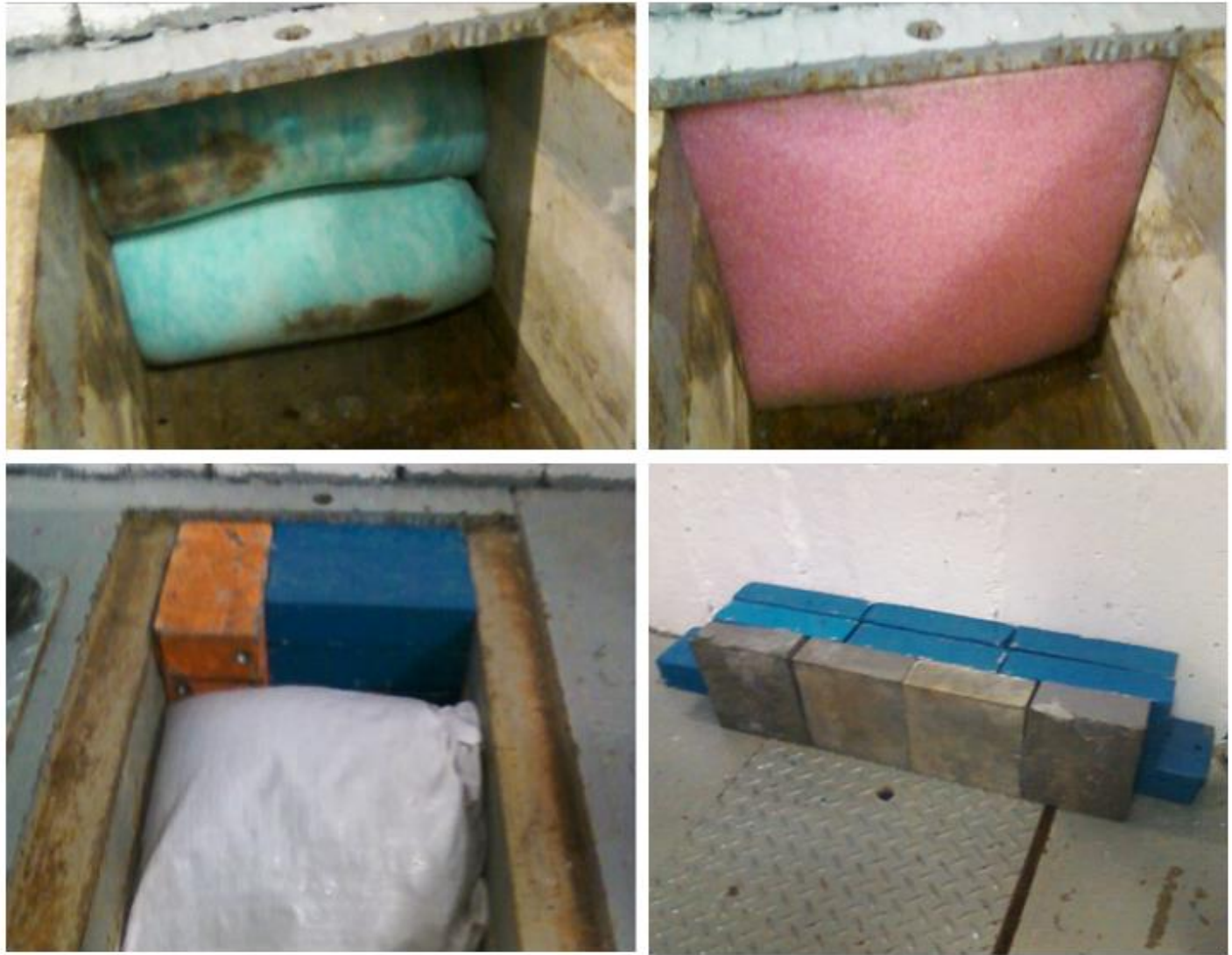
Figure 9: floor trench preparations to address ODH and radiation shielding concerns: the top images show foam installed inside the trench to restrict the flow of ODH gas, and the bottom images show lead brick and gravel-bag shielding inside the trench and lead brick above the iron trench plate. This shielding is a vital credited control and is under RCD control and cannot be removed without permission. Credited control signage is located at each trench, although not shown in the photos above.
