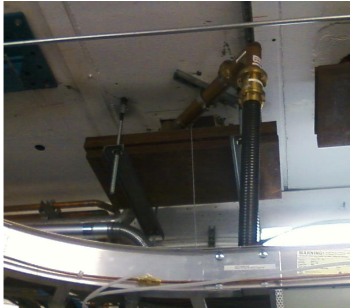
Figure 8: The rigid coaxial RF waveguide passing through a rectangular ceiling penetration in Cave 1, connecting the buncher cavity to the solid state amplifier. The iron plate hanging below the penetration provides radiation shielding.
