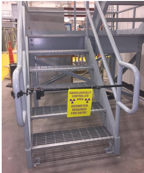
Figure 10: During UITF operations, the top of UITF Cave 1 roof is a Radiologically Controlled Area and dosimetry is required to access the roof.
