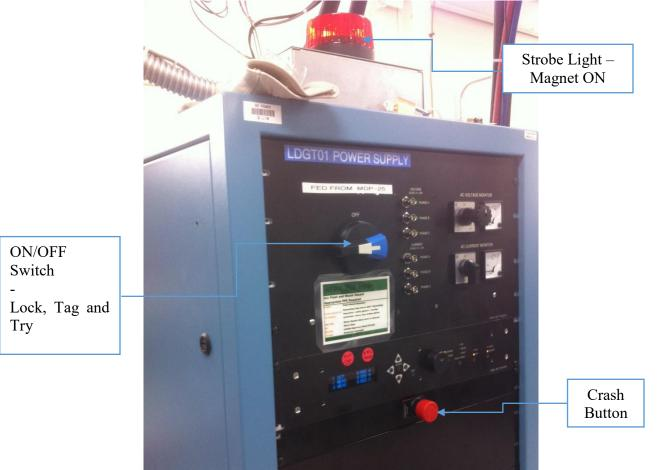
Figure 2: Magnet power supply at the GTS mezzanine. There is a crash button on the front panel.
