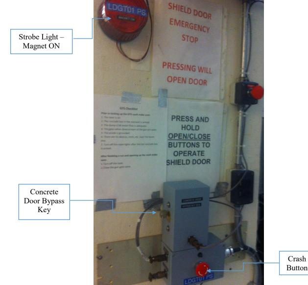
Figure 3: Magnetic field strobe light indicator at the access door. Also shown, the magnet power supply crash button.
