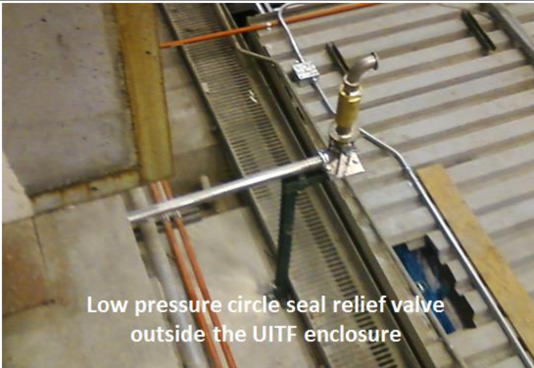
Figure 16: top left shows the three relief ports of the QCM vent stack. Top right shows the deflector sheet metal attached to the parallel-plate relief which would direct gaseous helium upward and not toward occupants inside the UITF enclosure. The bottom figure shows piping attached to the exhaust port of the circle seal relief which would direct vented gas out of the UITF enclosure.
