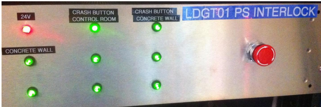
Figure 5: Cathode magnet power supply interlock box in the GTS Control Room (Rack GL01B15)
