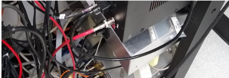
Figure 4: IA system HV supply and switch used at CEBAF laser table.
