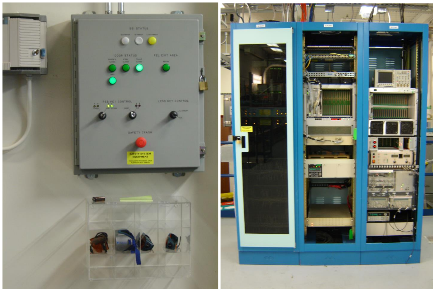
Figure 5: (Left) PSS console is located in the GTS control room. (Right) PSS rack is located in the GTS mezzanine alongside racks housing IOCs, controls and monitoring equipment.
