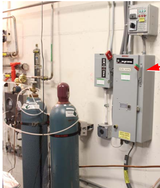
Figure 3-1: Gun HV Power Supply Disconnect Switch
