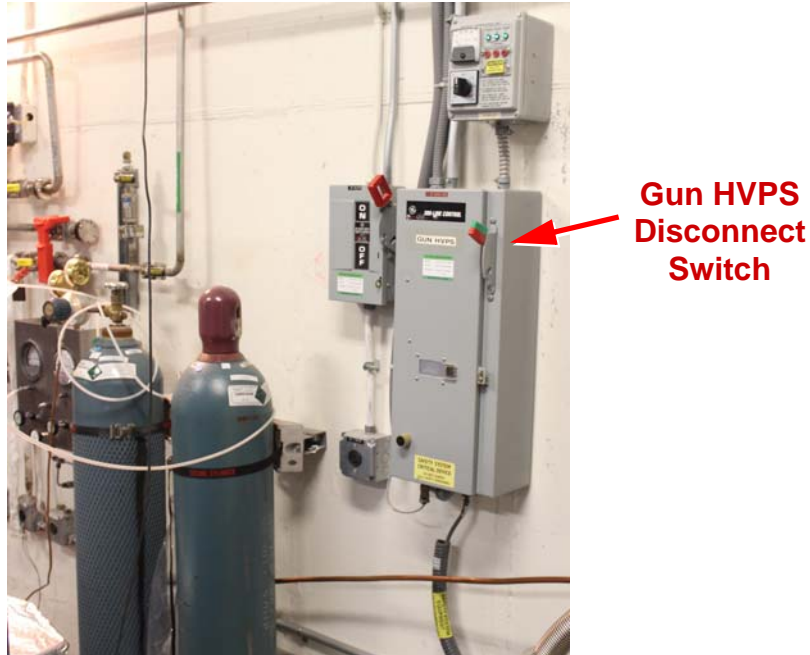
Figure 4-1: Gun HV Power Supply Disconnect Switch
