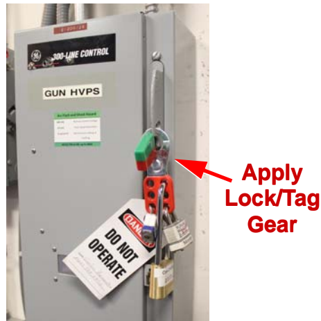
Figure 3-3: Apply Lock/Tag
