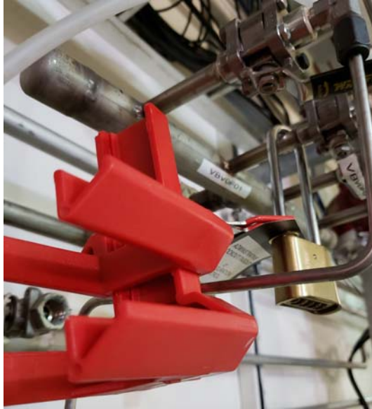
Figure 2-1: Lock/Tag Gear Locked to Air Supply Line for Storage
