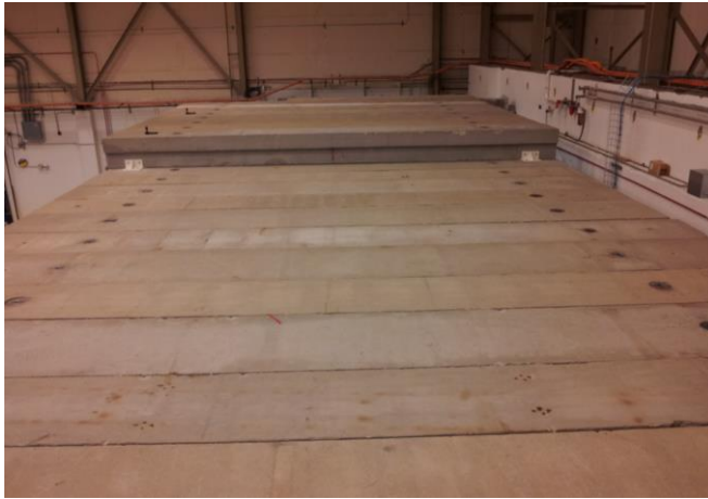
Figure 9 (Left) Shielded elevated-roof section of Cave 2, which will be used for experimental targets, including cryogenic targets. (Right) 5.6 m 2 Vent area beneath the elevated roof section of Cave2, for lighter than air cryogenic gases to escape.
