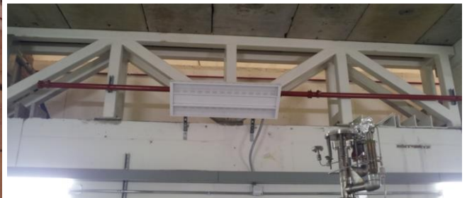
Figure 9 (Left) Shielded elevated-roof section of Cave 2, which will be used for experimental targets, including cryogenic targets. (Right) 5.6 \text{ m}^2 Vent area beneath the elevated roof section of Cave 2, for lighter than air cryogenic gases to escape.
