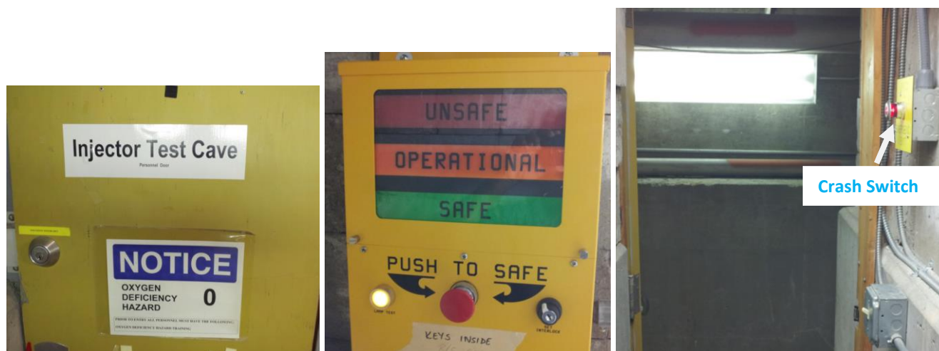
Figure 7 (Left) Exit into high bay from Cave 1 near the electron gun (Middle) Run/Safe Box (Right) Crash Switch for exit. Run/Safe Boxes and Crash switches are at both the entrance/exit ways
