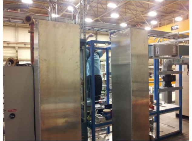
Figure 8 (Left) Fan with a capacity of 7400 CFM vents air into the high bay area, (middle) fan with a capacity of 4400 CFM vents air to outside the test lab, right two chimneys attached to the square vent holes in the ceiling of Cave 1
