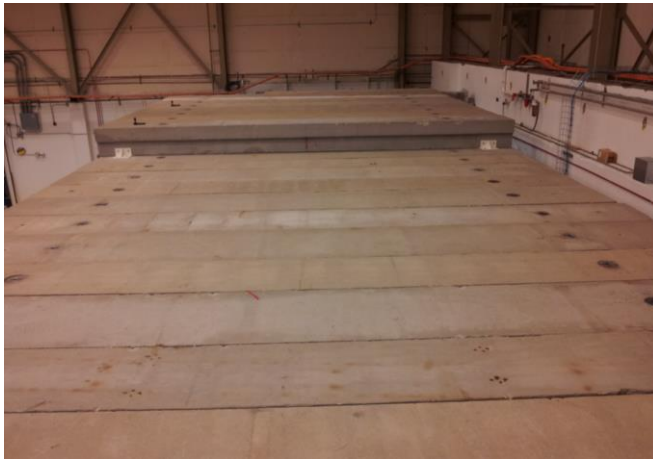
Figure 9 (Left) Shielded elevated-roof section of Cave 2, which will be used for experimental targets, including cryogenic targets. (Right) 5.6 \text{ m}^2 Vent area beneath the elevated roof section of Cave 2, for lighter than air cryogenic gases to escape.
