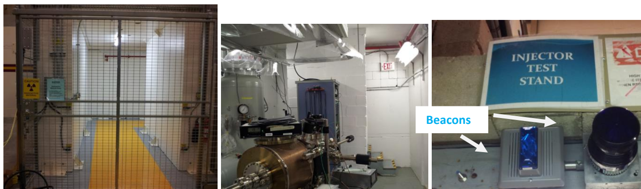
Figure 6 (Left) Main entrance/exit from high bay area through the labyrinth of UITF (Middle), Secondary exit into the high bay from the southern-most location of the keV section. Both doors have Personnel Safety System interlocks and emergency exit switches on the nearby walls (Right). Beacons exist at both entrance/exit ways
