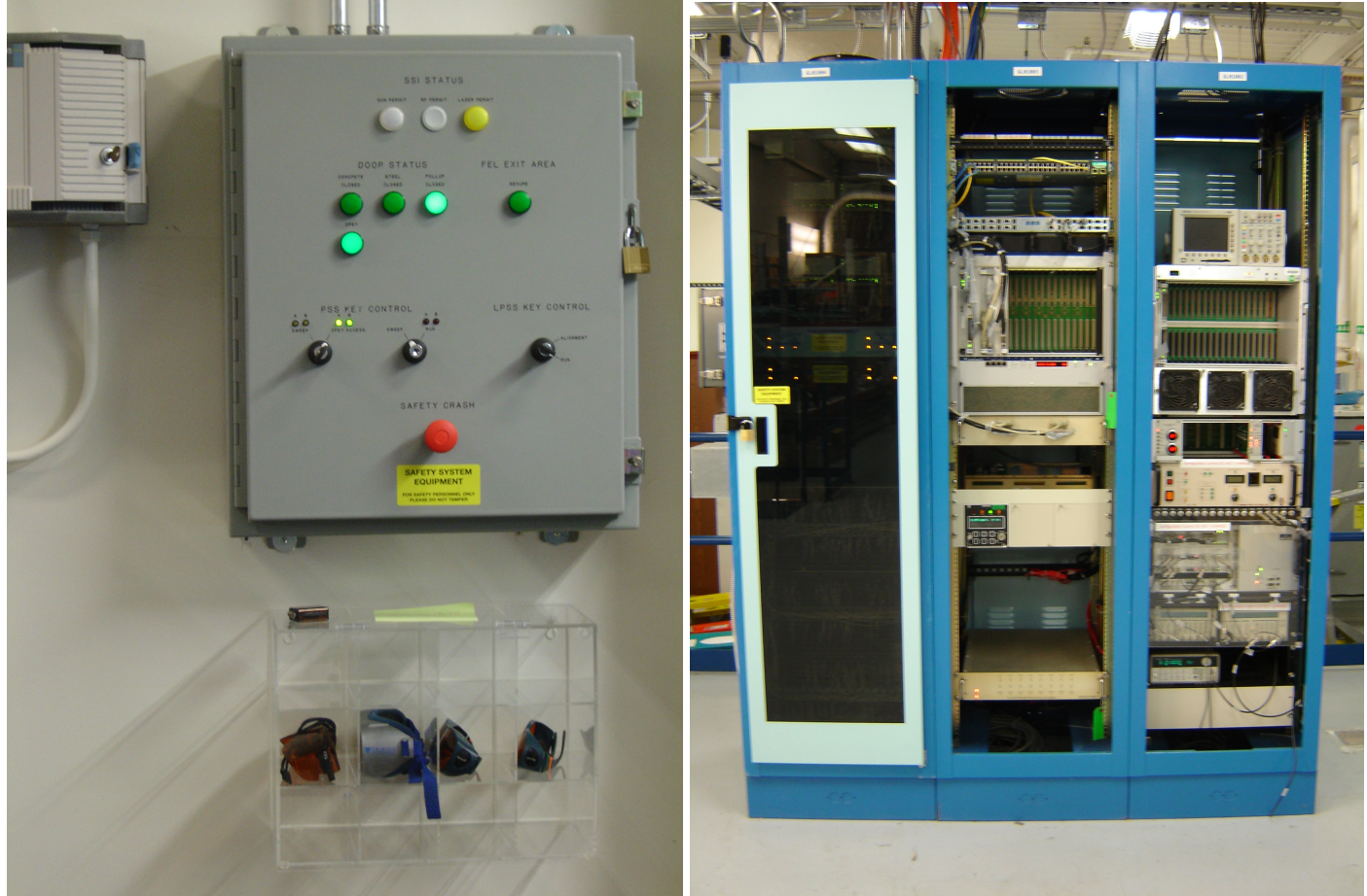
Figure 6. Left, the PSS console is located in the GTS control room. Right, the PSS rack is located in the GTS mezzanine alongside racks housing IOCs, controls and monitoring equipment.
