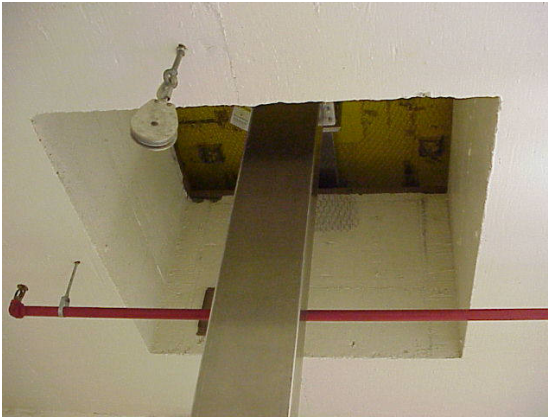
2 nd Floor 4x4 Ceiling Vent, West End
