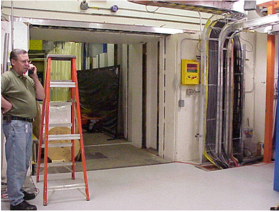
1 st Floor Main Lift Door/Floor Trench
