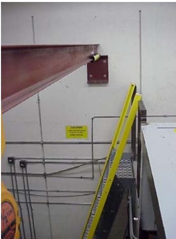
2 nd Floor Stairway
