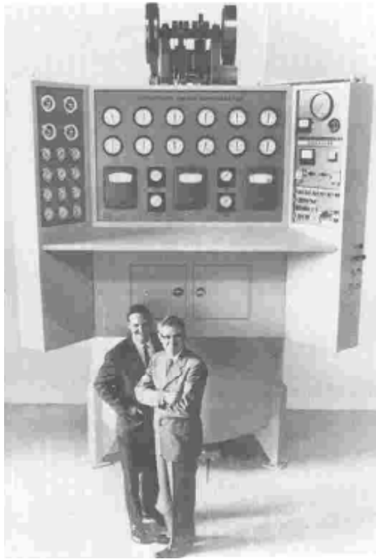
Figure 7.2.1: Stanford University 300W, 1.8 K Helium Liquefier (1969)
