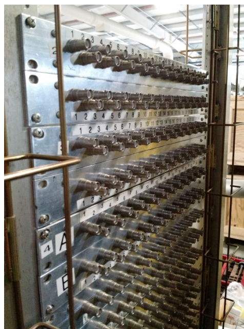
High density HV breakout panel (BETA weldment in ESB)
