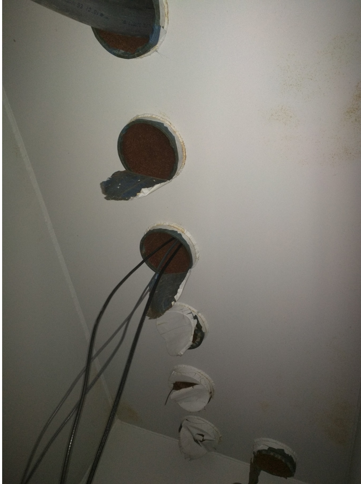
Penetrations into SHMS electronics hut
