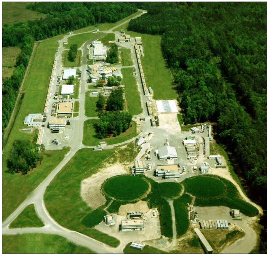
Fig. 1. Aerial photograph of the JLab site. Hall A is the leftmost circular mound in the lower part of the figure. For scale, the diameter of Hall A is 52 m.
